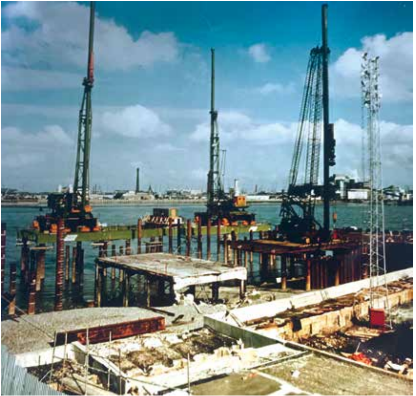
Fig 25. 1976 Piling for Pier 9 and South Abutment
