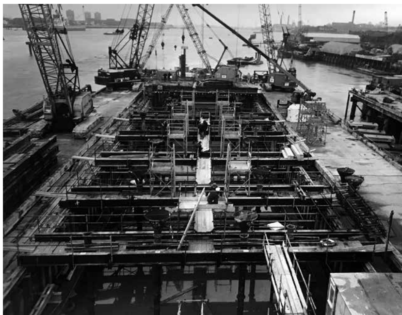
Fig 27. 1976 Preparing for underwater concrete
