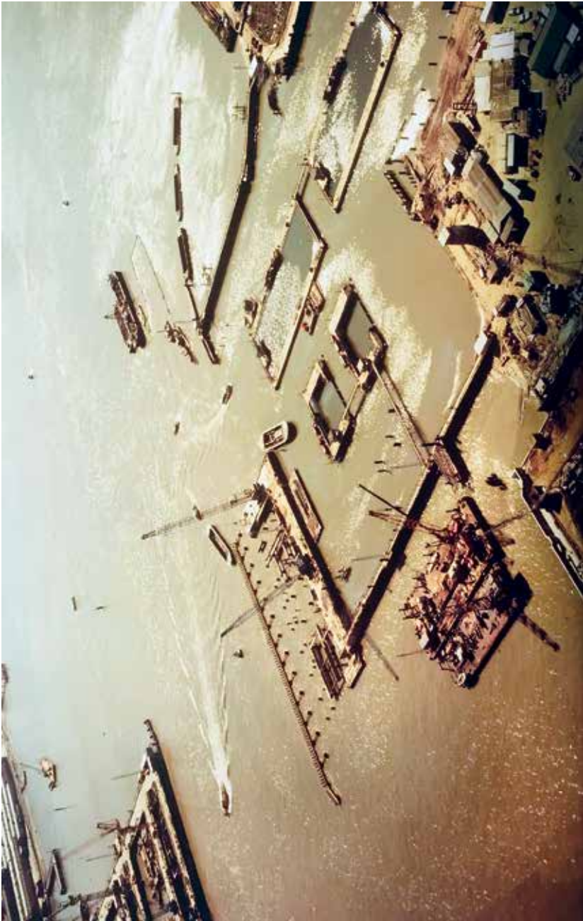
Fig 41. 1977 Flooding north dry dock for sill tow out
