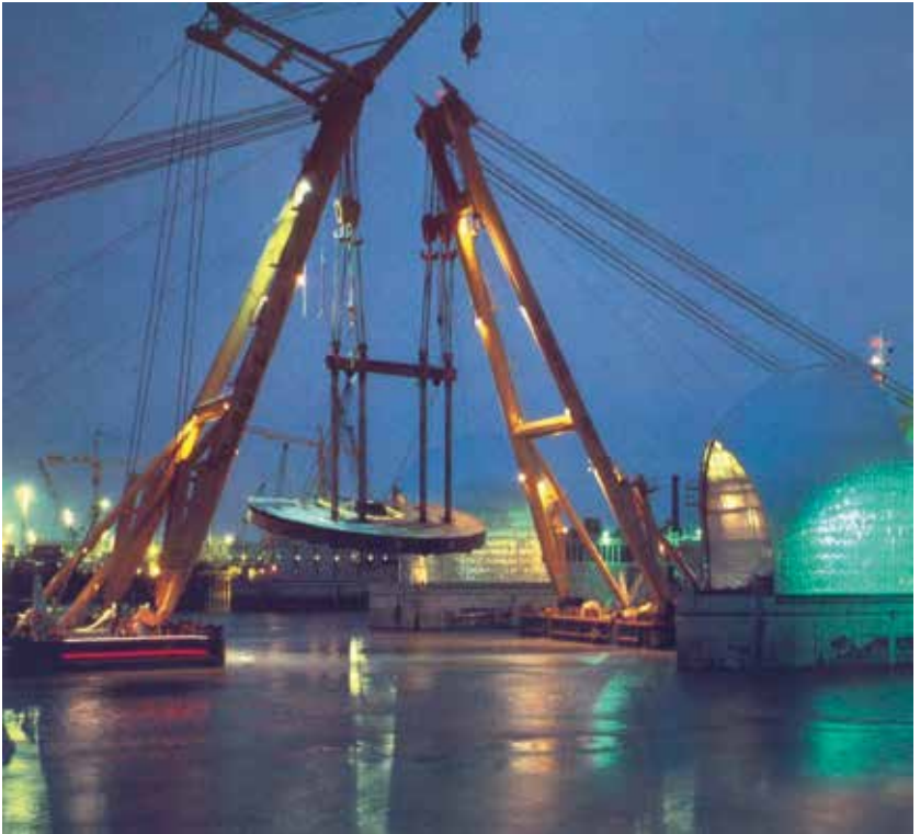
Fig 56. Placing the Gate Arm
