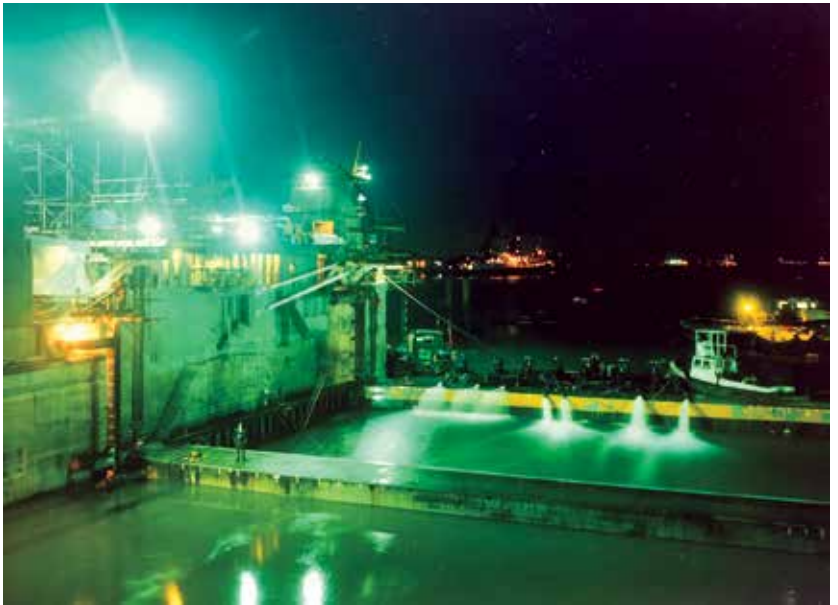
Fig 45. Water filling of sill scallop before lowering
