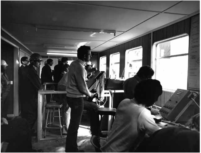
Fig 44. Sill lowering, control cabin
