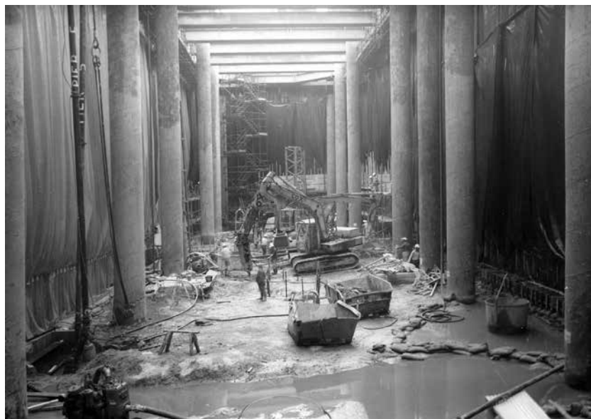
Fig 28. Clearing laitance on surface of underwater concrete
