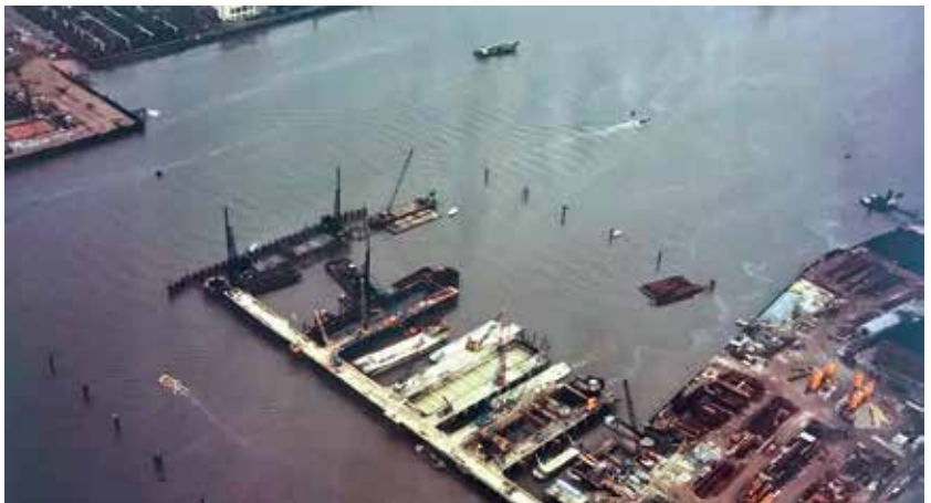
Fig 26. 1976 Completing Cofferdams and Excavation of Piers 6-9
