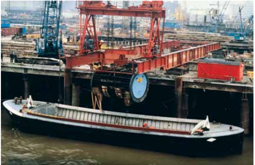
Fig 30. Lifting the Trunnion into Pier 4
