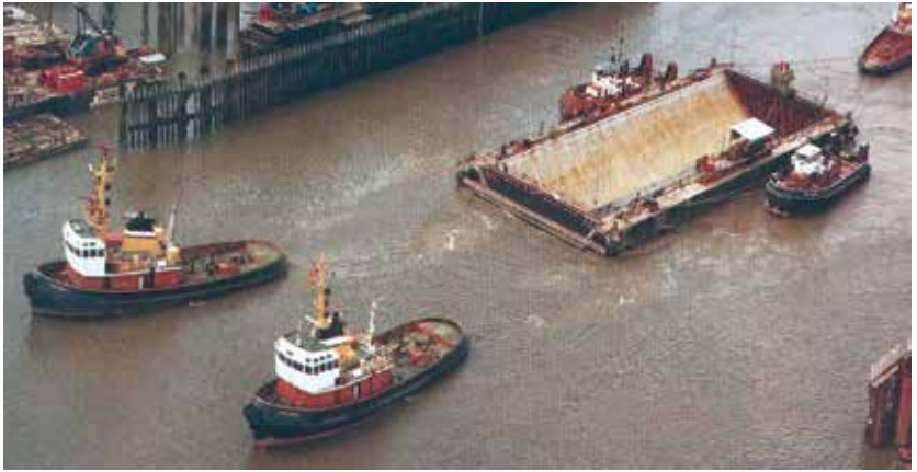
Fig 42. Sill Tow out from George V dock
