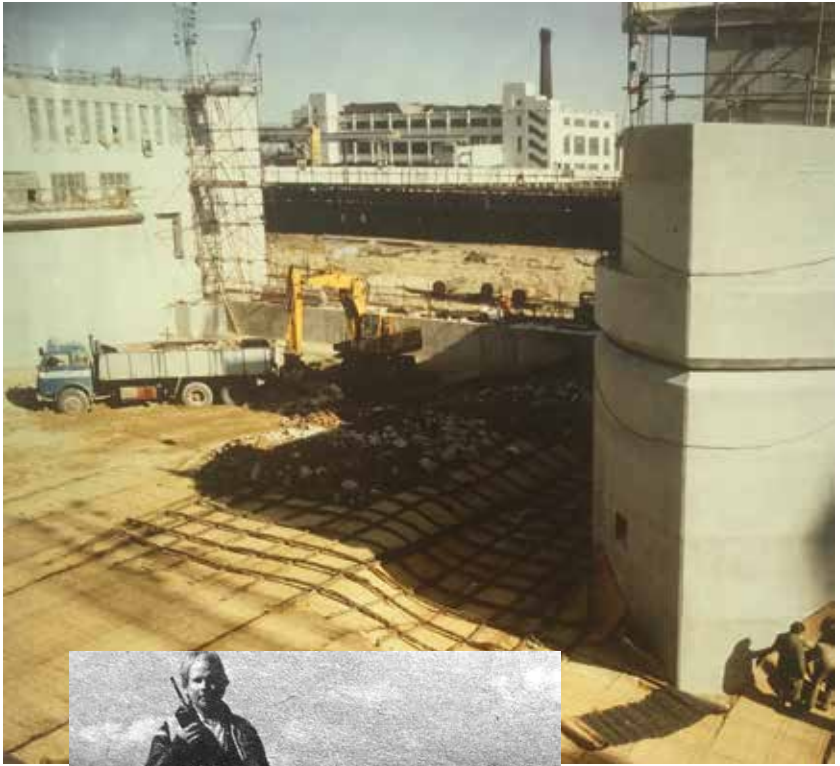
Fig 59. Placing Bed Protection between Pier 1 and Pier 2
