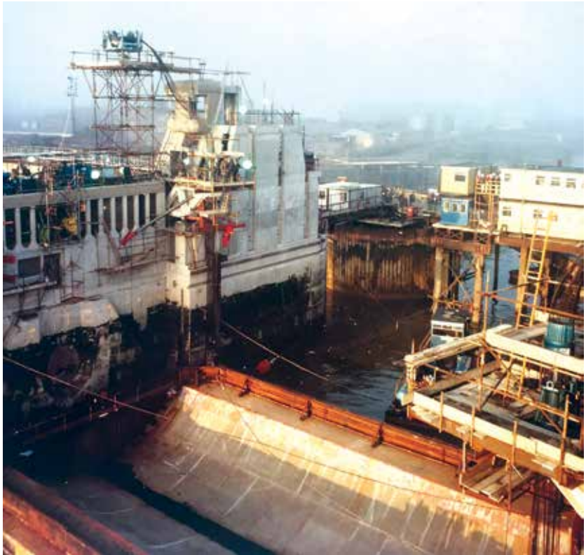
Fig 43. Sill positioning at the pier
